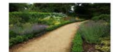
Precedent of Decomposed Granite Pathway A decomposed granite pathway is better for drainage as decomposed granite is a permeable material. It easy to maintain, helps prevent erosion, minimizes flooding, and is overall a more ecologically sustainable option than asphalt for this site.
