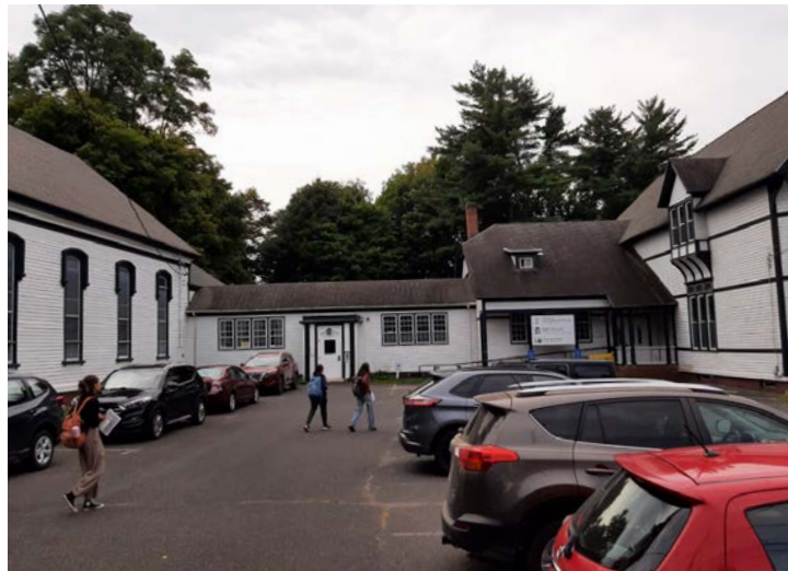
The parking lot in front (north) of the building, which may be converted into a pedestrian plaza.
